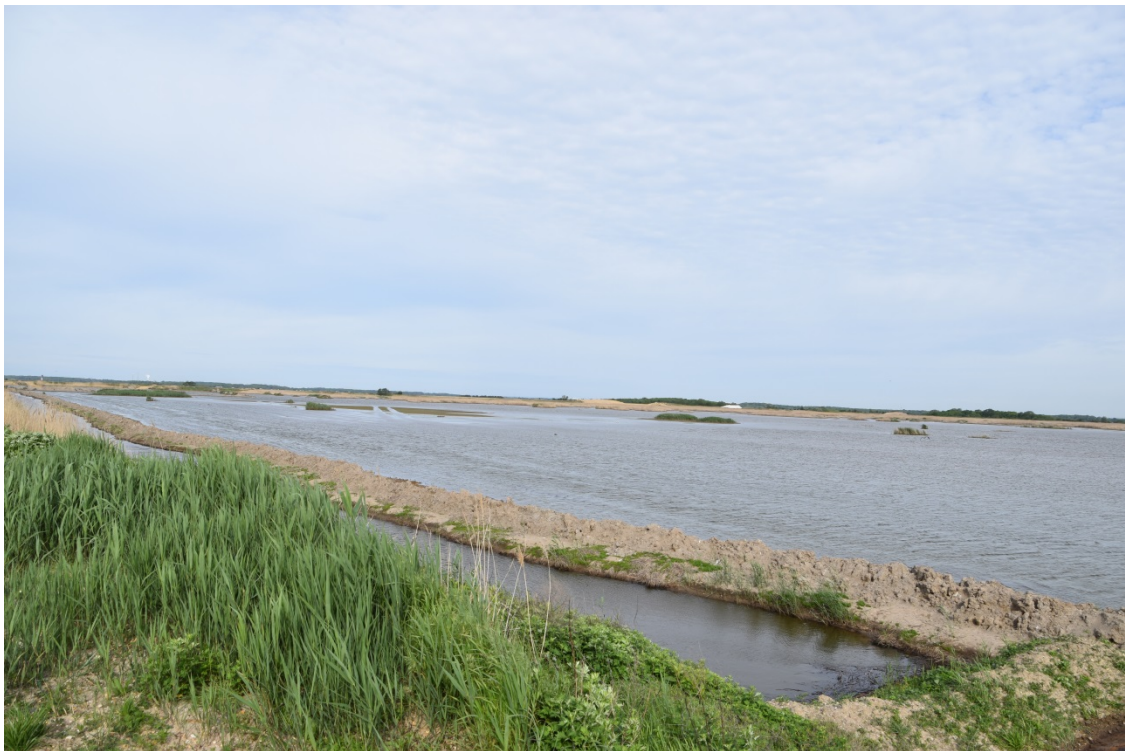
Spillway 009, looking southwest
