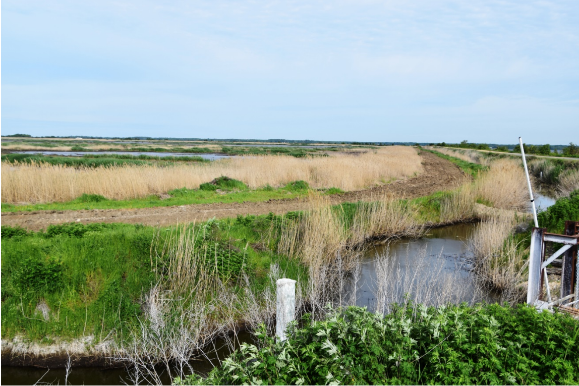
Spillway 007, looking east
