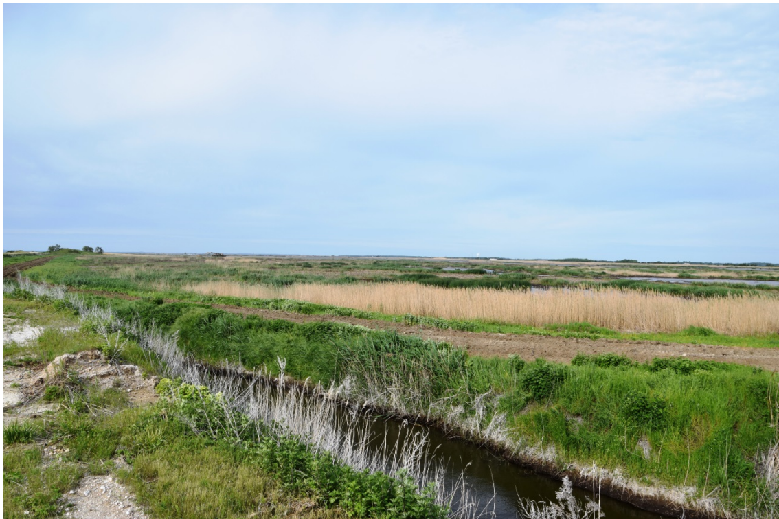
Spillway 007, looking west
