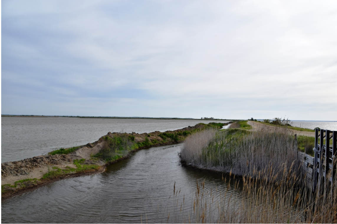
Spillway 009, looking northeast
