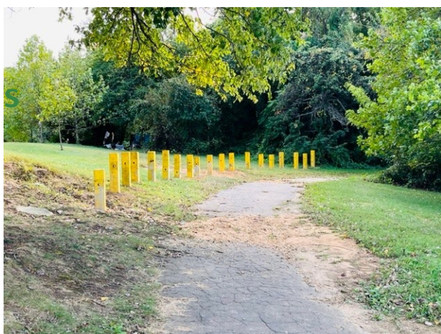
Used wharf logs installed along the park's edge. Photo by Dan Spack/EcoLogix Group
