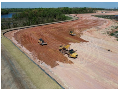
Base Dike Widening at Cox Creek DMCF. Photo by MPA
