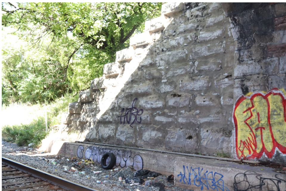
Photo 4: Detail of west portal abutments, looking northwest
