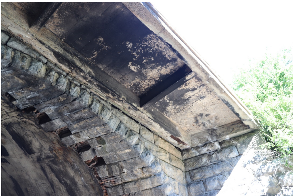
Photo 6: Underside of the 1914 decking expansion, looking northwest
