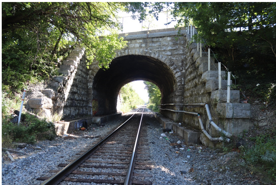
Photo 2: West portal, looking east
