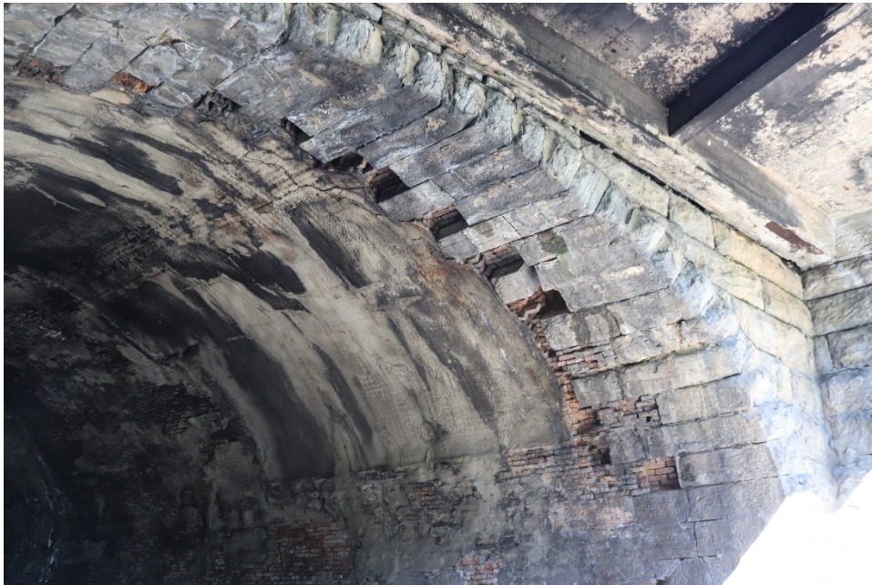
Photo 5: Interior Brick and Concrete Lining, Looking Northwest
