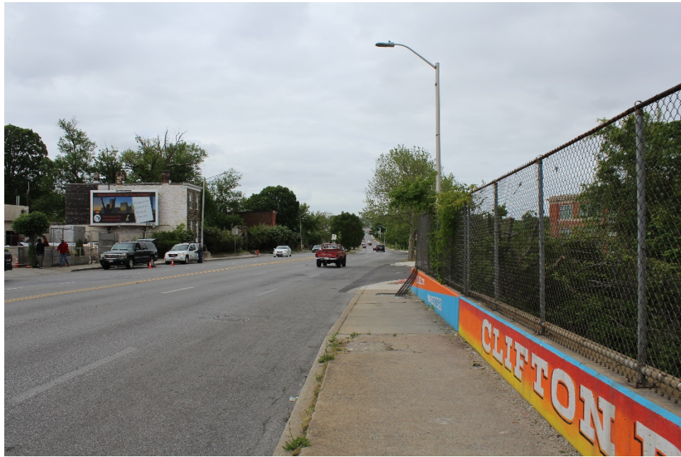
Photo 7: Harford Road over CSX tracks, looking northeast
