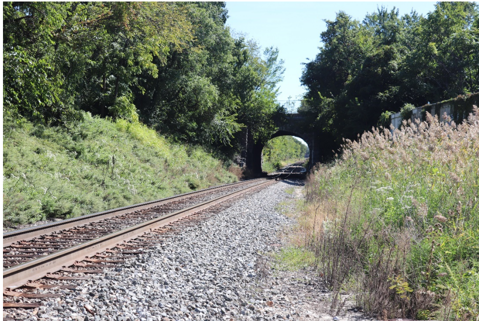
Photo 1: West portal, looking east
