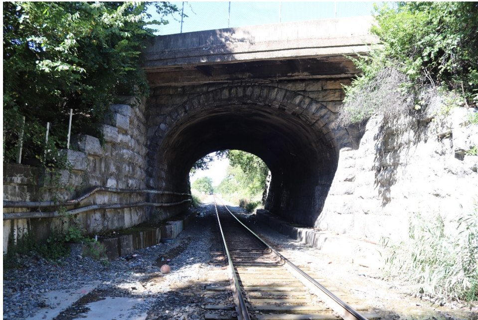
Photo 3: East portal, looking west
