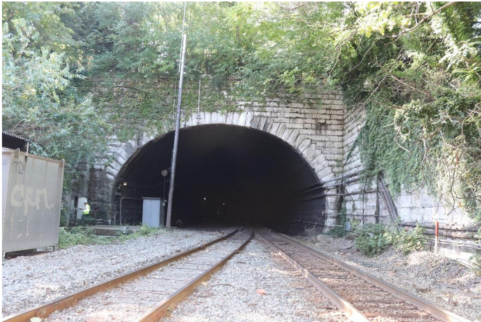
Photo 2: North portal, looking south
