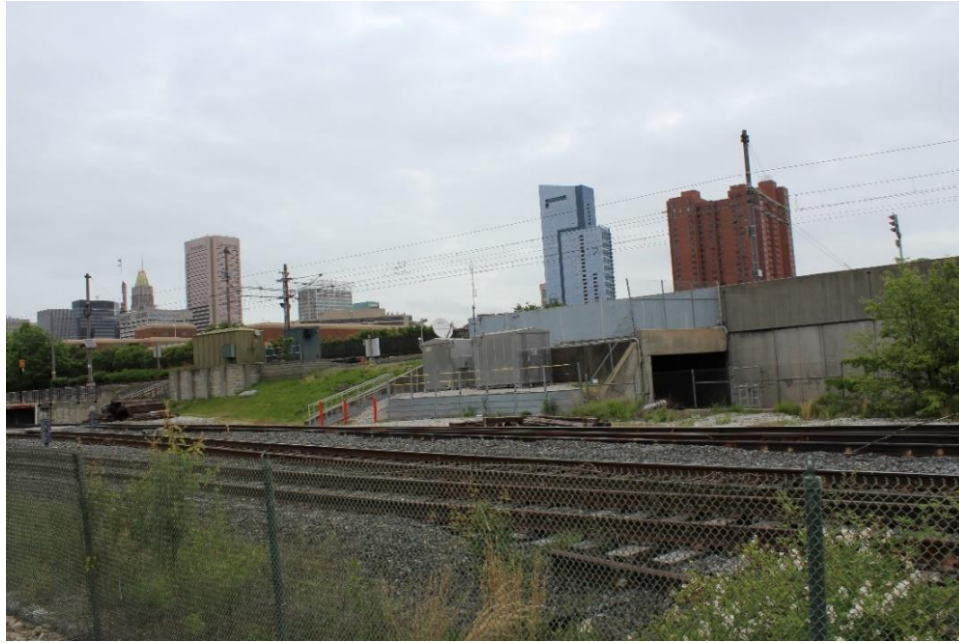
Photo 19: South portal, looking northeast from parking lot north of Martin Luther King Jr. Boulevard
