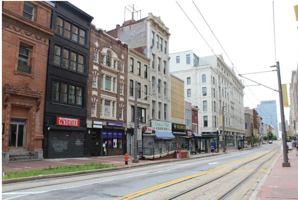
Photo 21: Howard Street with the Howard Street Tunnel below ground, looking south at West Saratoga Street
