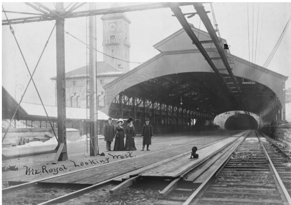
Historic Image 2: Mount Royal Station, looking southeast toward the north portal of the Howard Street Tunnel, late nineteenth century. Photo credit: B&O Railroad Museum.
