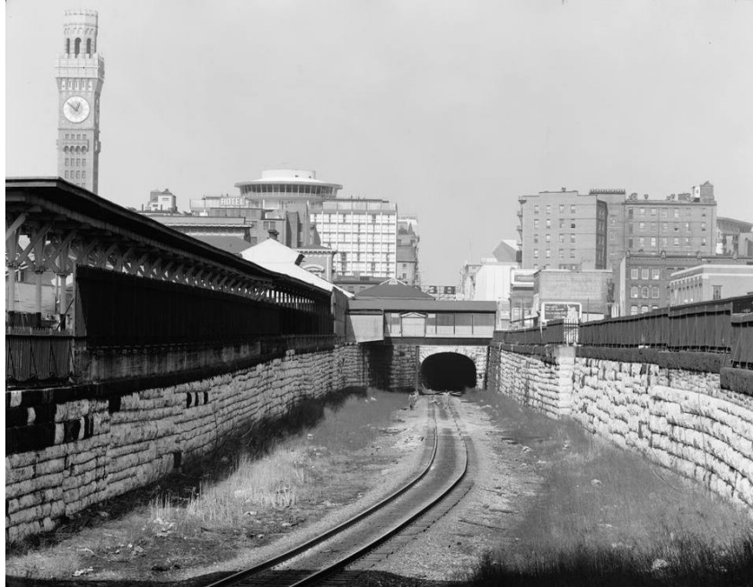
Historic Image 5: The former south portal at Camden Station, which was enclosed for the construction of I-395, 1971. Photo Credit: Historic American Engineering Record, Library of Congress.
