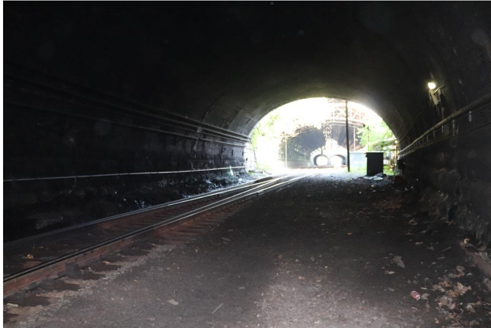
Photo 9: View from tunnel, looking north to trainshed at Mount Royal Station
