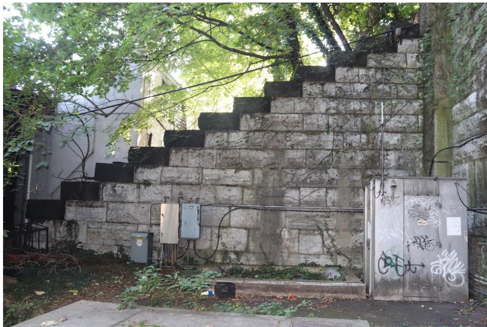
Photo 4: North portal abutment, looking east
