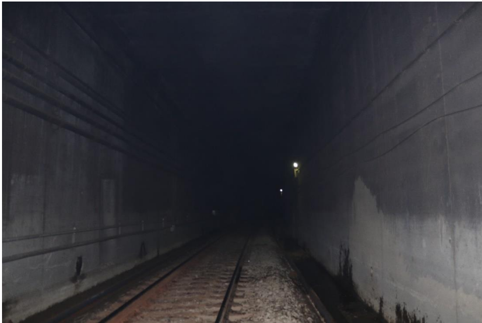
Photo 16: View within tunnel, looking north from the 1982 boxed concrete section
