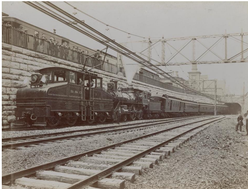
Historic Image 4: Spectators watch as an electric locomotive pulls a steam locomotive and railcars at south portal of the Howard Street Tunnel, ca. 1895. Photo Credit: The Maryland Center for History and Culture, Item MC4171.1.
