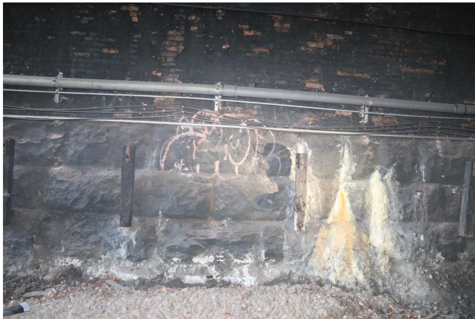
Photo 6: Typical side wall view, looking east near Mount Royal Station
