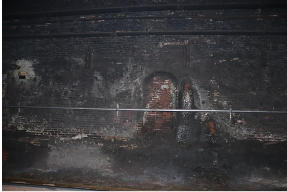
Photo 7: Typical pedestrian safety alcove, looking west near Mount Royal Station
