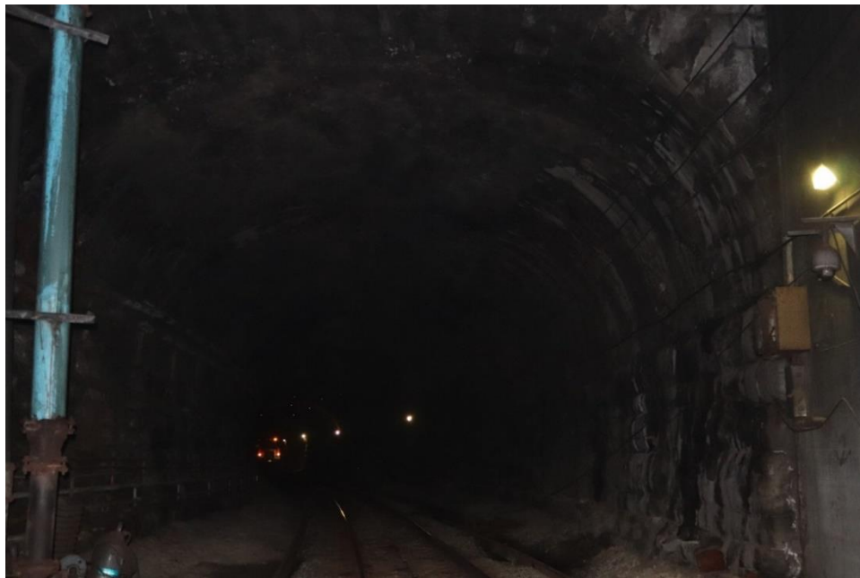
Photo 14: View within tunnel, looking north at the junction of the 1895 south portal and the boxed concrete section
