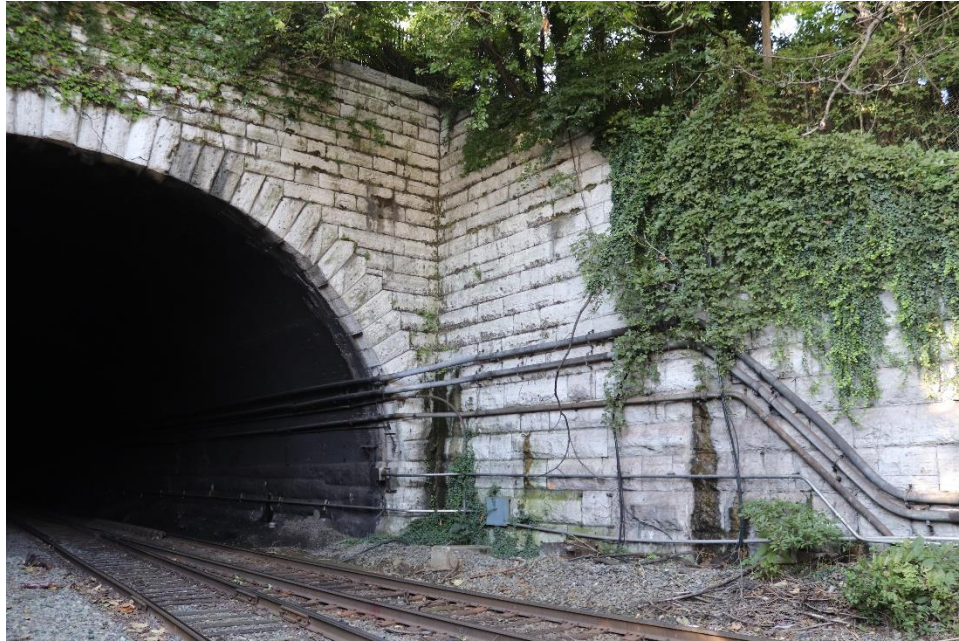
Photo 3: North portal and abutment, looking southwest
