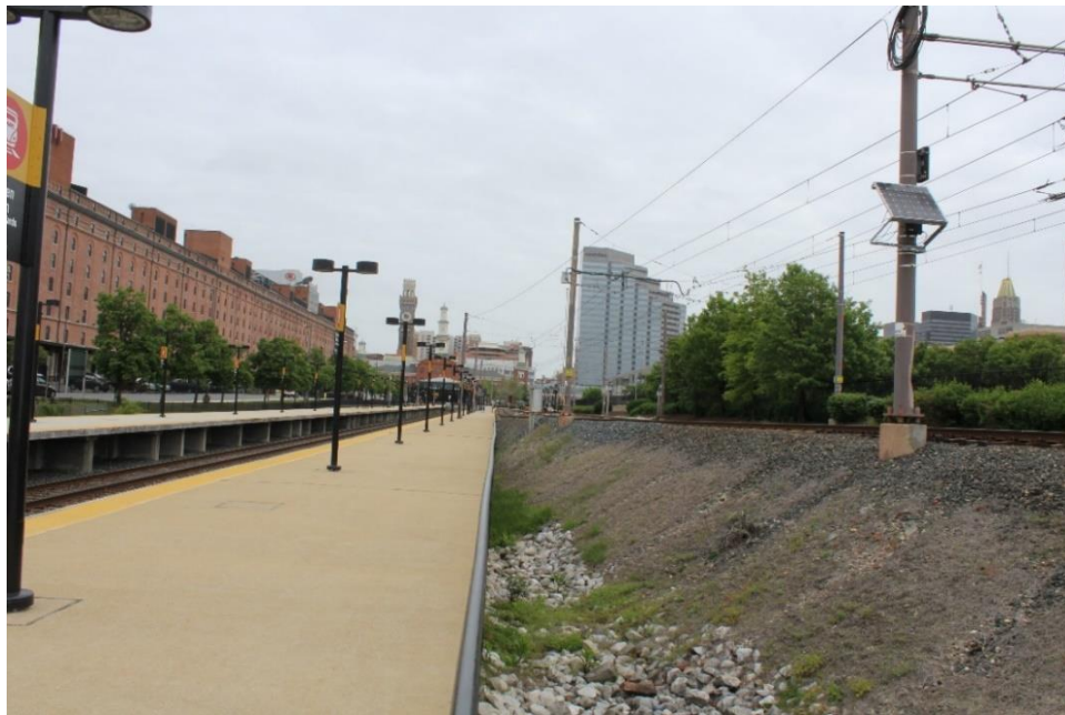
Photo 20: B&O Railroad warehouse and Camden Station, looking north to Howard Street; former B&O Railroad siding now used by MARC seen at left, MDOT MTA light rail tracks at right, with the Howard Street Tunnel below ground
