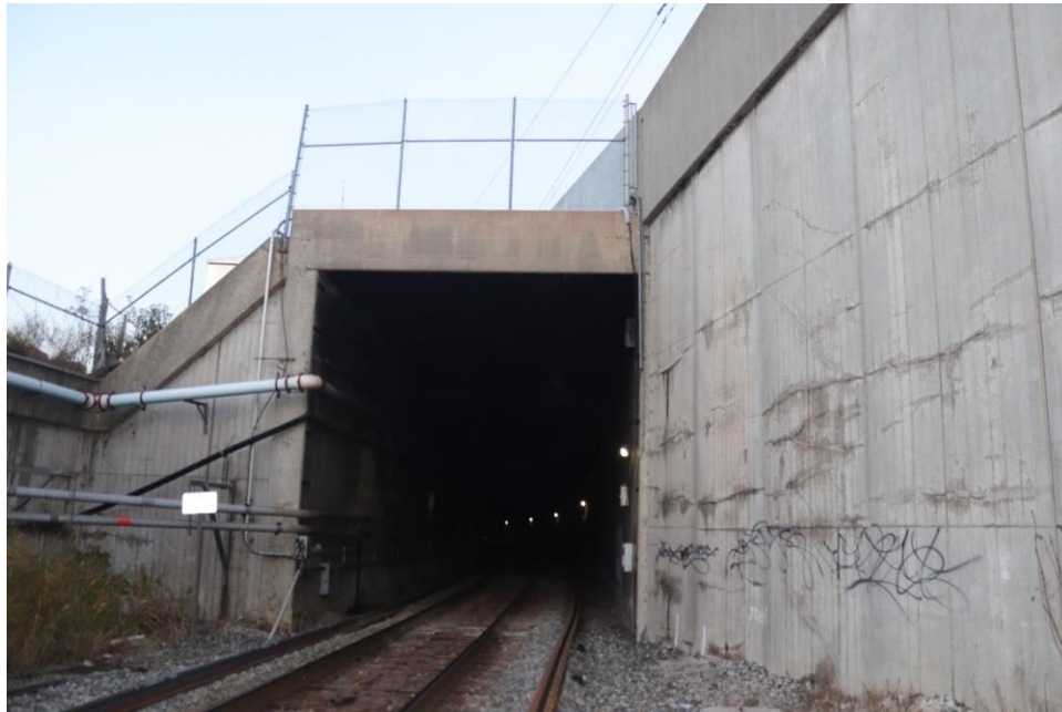
Photo 17: South portal, looking north
