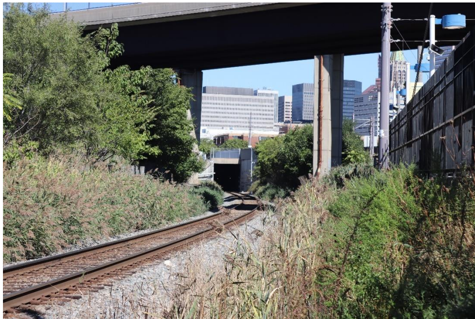
Photo 18: South portal, looking north from beneath Martin Luther King Jr. Boulevard
