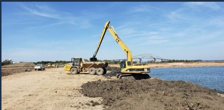
*Photo: During the innovative reuse material drying operation, material excavated from the DMCF is placed on set drying pads to dry prior to stockpiling for reuse.
