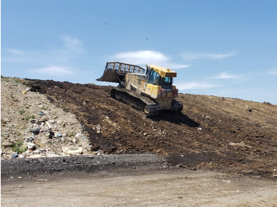
In December 2018, MDOT MPA provided approximately 6,000 cubic yards of dewatered dredged material from Cox Creek DMCF for use as ADC at the Baltimore City-owned Quarantine Road Landfill. To date, 3,000 cubic yards have been used. Photo by MDOT MPA
