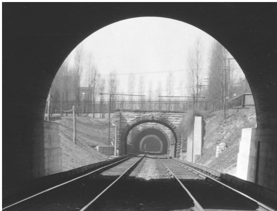
Figure 3: East portal of the B&O Railroad Guilford Avenue Tunnel, looking west from the Barclay Street Tunnel, ca. 1925. The east portals of the St. Paul and Calvert Street and the North Howard Street, Maryland Avenue, and North Charles Street Tunnels can be seen in the background. (Image courtesy of the B&O Railroad Historical Society.)
