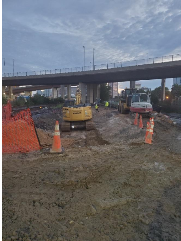
Figure 3: Stormwater Management Detention Basin Project Area. Hydric subsoils exposed in base of excavation.
