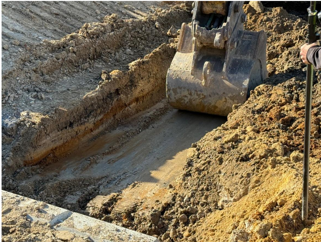
Figure 3: Stormwater Management Detention Basin Project Area. Hydric subsoils exposed in base of excavation.
