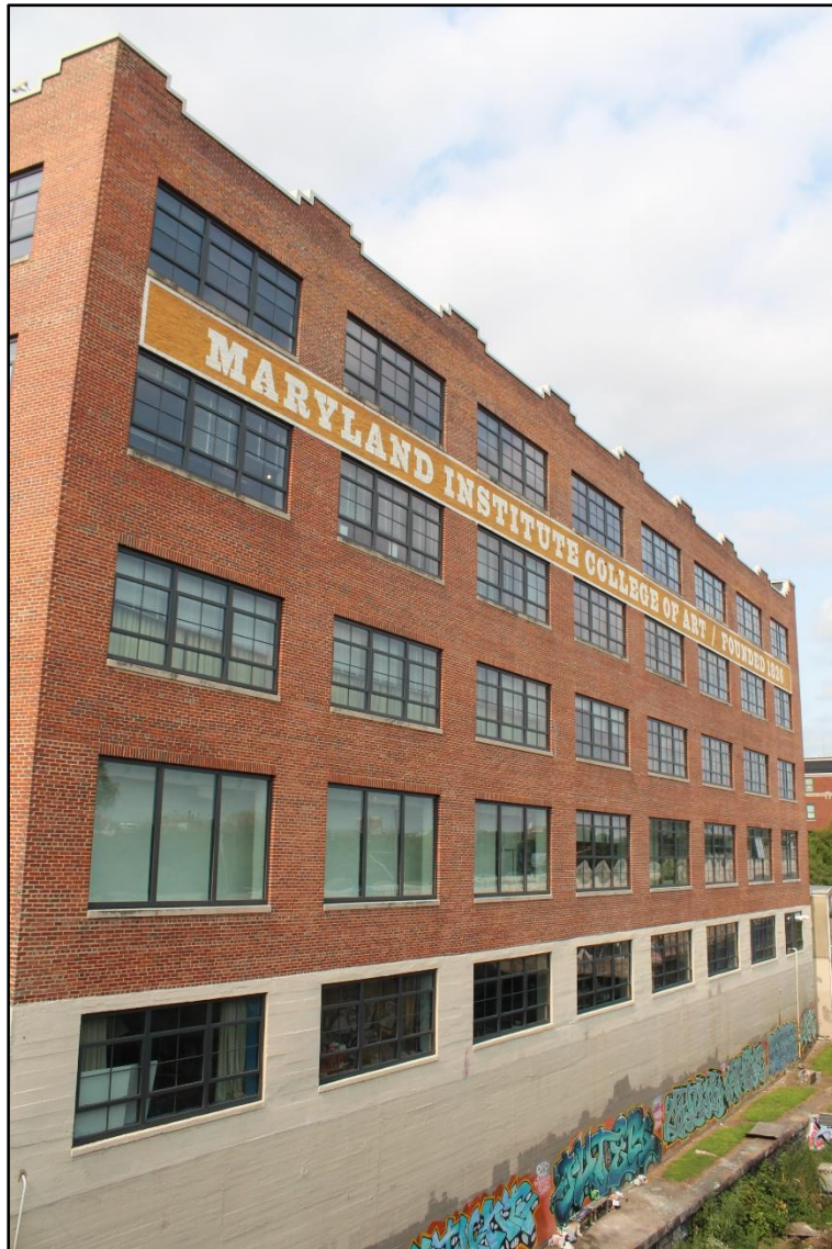
Photo 4: Northeast elevation, facing northwest
