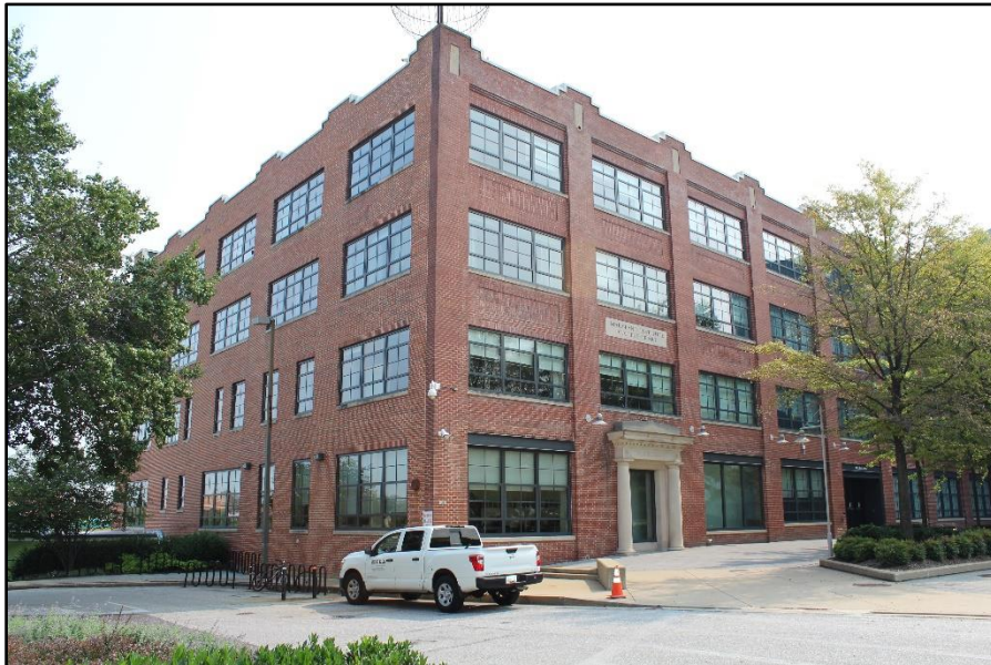
Photo 1: Southwest façade and northwest elevation, facing east
