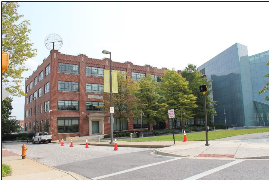
Photo 2: Southwest façade and attached Brown Center, facing east
