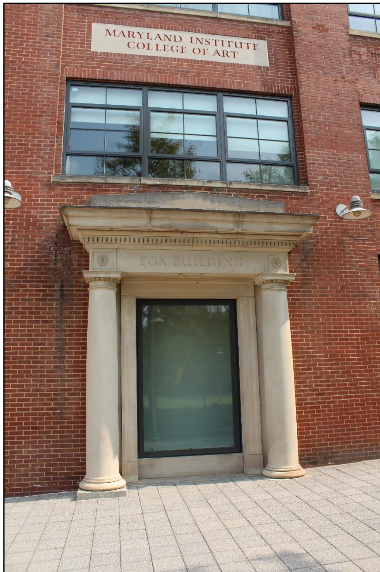
Photo 5: Detail of former entrance on the southwest façade, facing northeast
