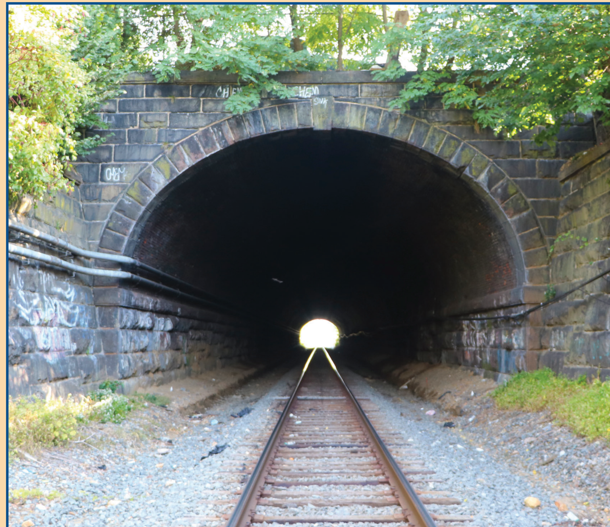
Boone Tunnel southwest portal and retaining walls, looking northeast. October 15, 2021.
