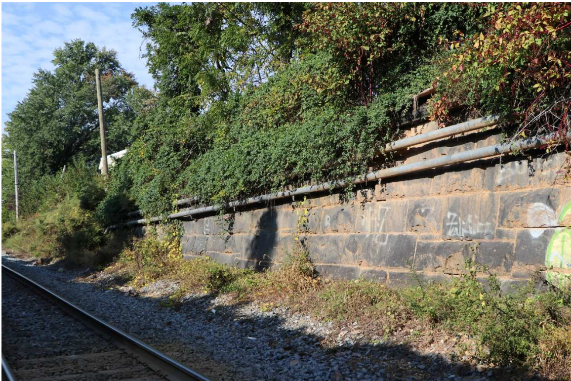
Photograph #11: Boone Tunnel northwest retaining wall, looking west. October 15, 2021.
