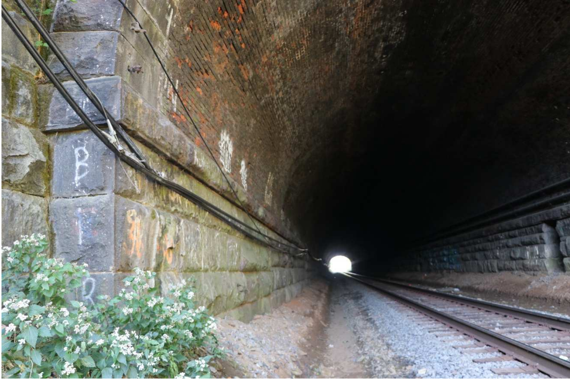
Photograph #5: Boone Tunnel interior view from northeast portal, looking southwest. October 15, 2021.
