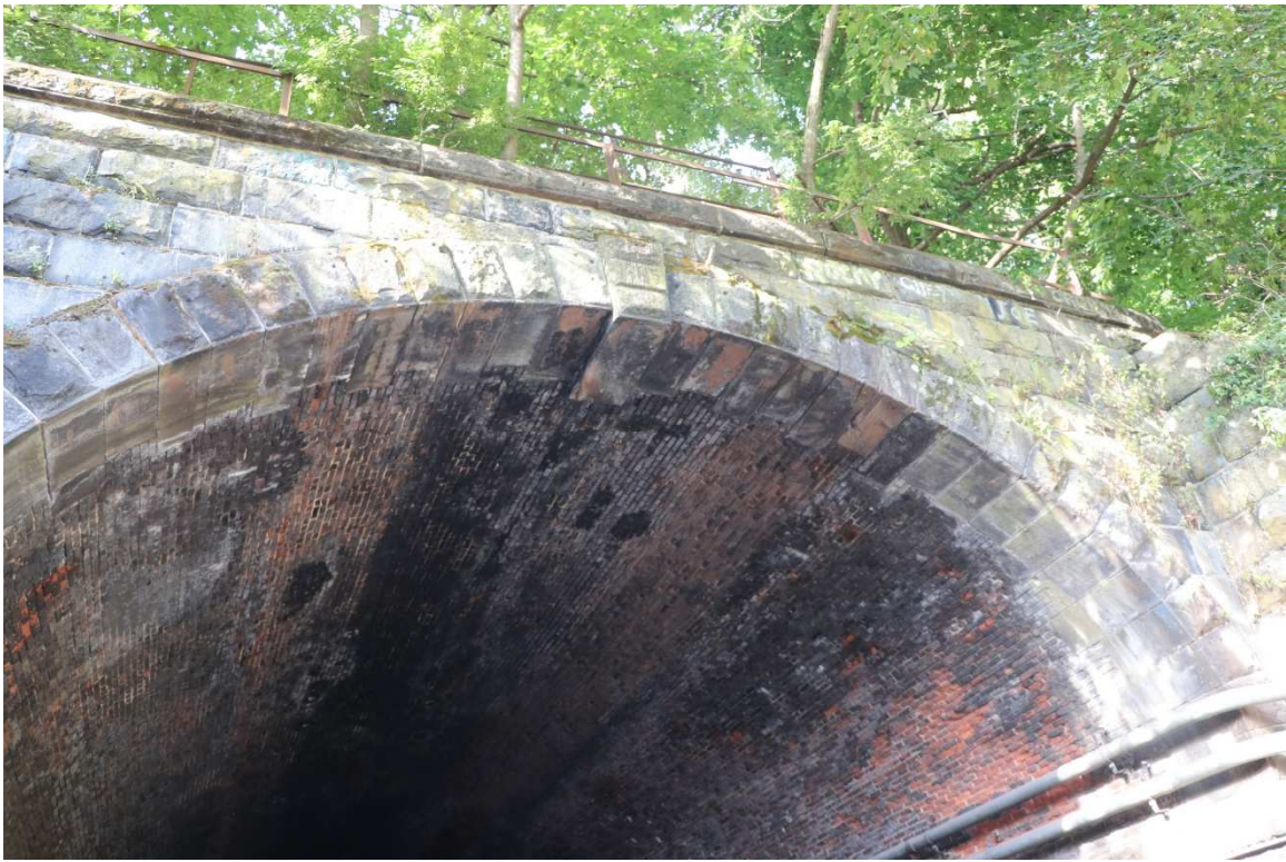
Photograph #6: Boone Tunnel northeast portal arch interior, looking southwest. October 15, 2021.
