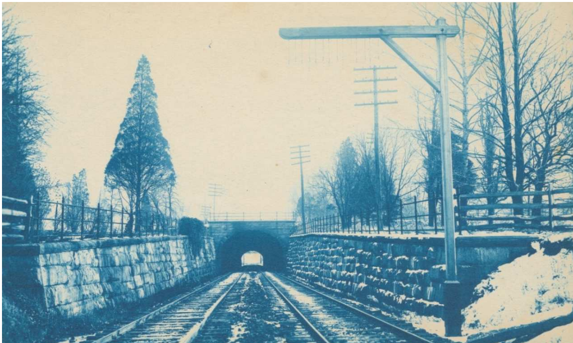
Boone Tunnel, southwest portal, looking northeast, March 1891 (Photo courtesy of the Library Company of Philadelphia)
