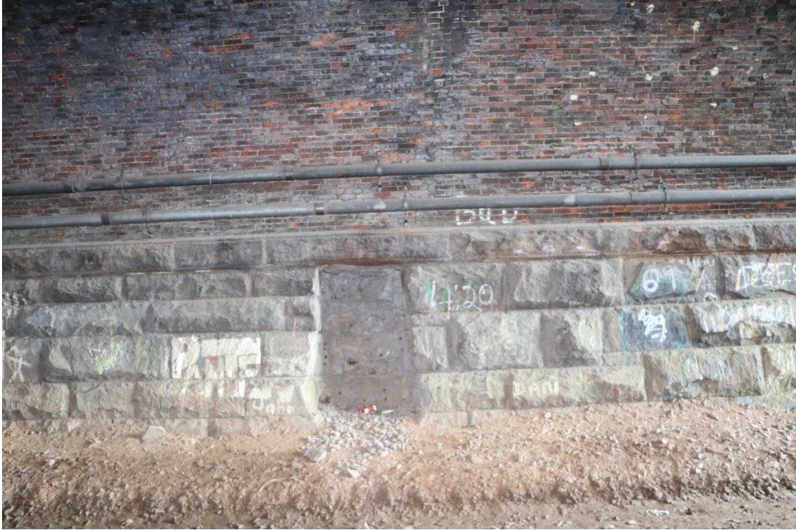
Photograph #10: Boone Tunnel interior, north wall, looking north. October 15, 2021.
