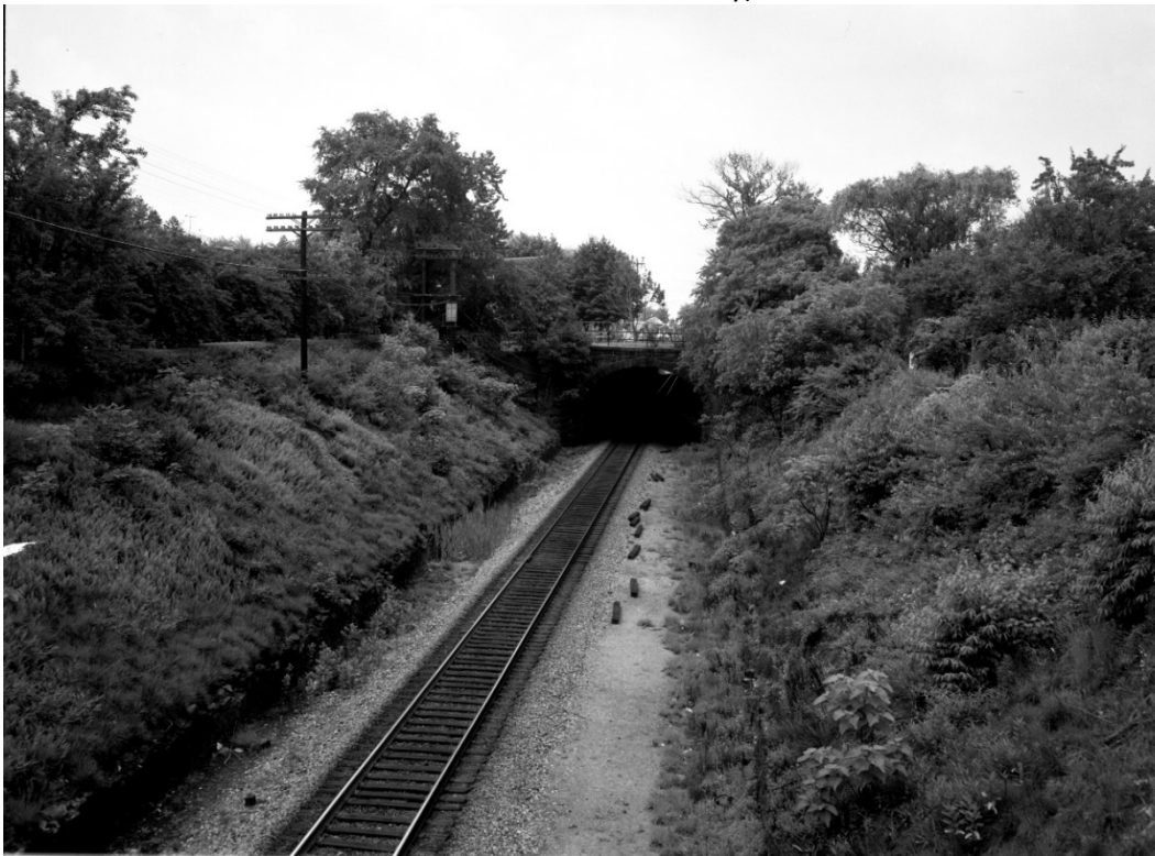
Boone Tunnel, northeast portal, looking southwest, June 1965 (Photo courtesy of the B&O Railroad Historical Society)
