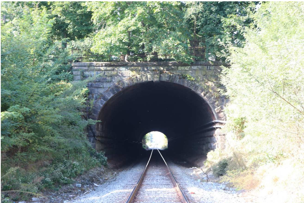
Photograph #2: Boone Tunnel northeast portal looking southwest. October 15, 2021.
