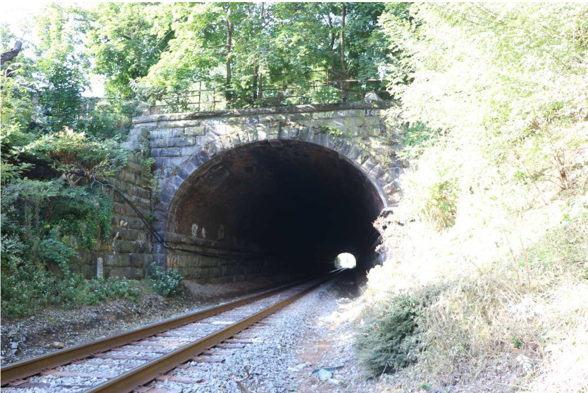
Photograph #4: Boone Tunnel northeast portal and retaining walls, looking southwest. October 15, 2021.
