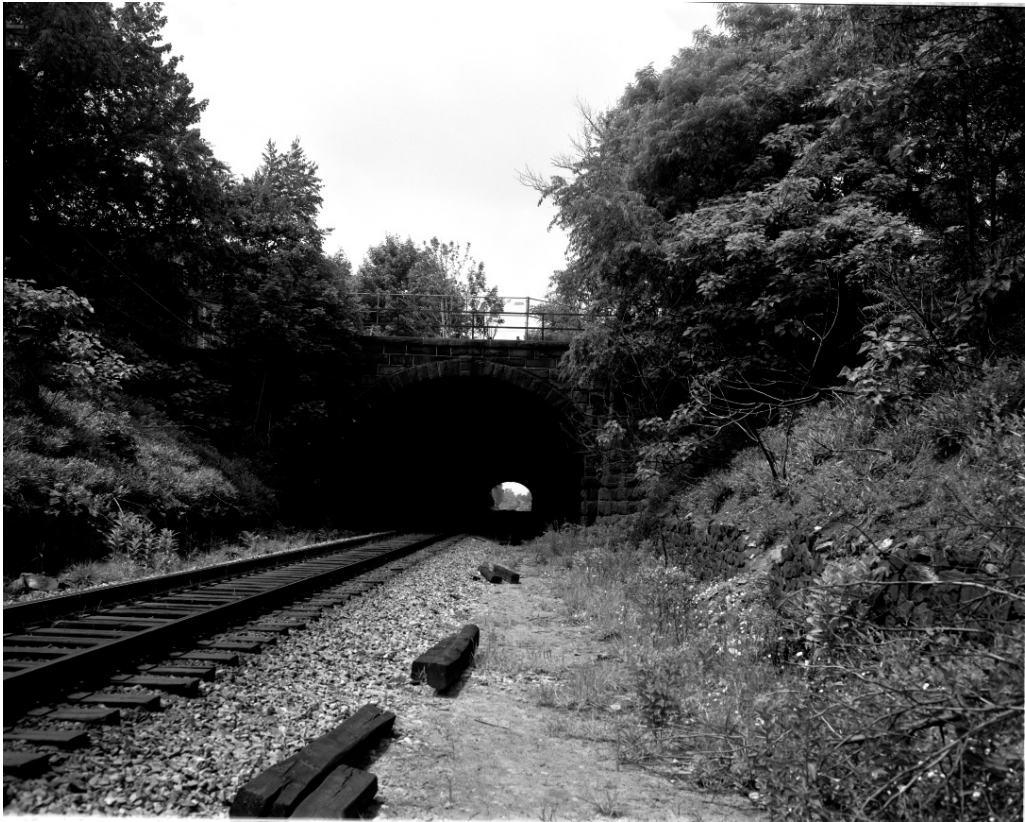
Boone Tunnel, northeast portal, looking southwest, June 1965 (Photo courtesy of the B&O Railroad Historical Society)
