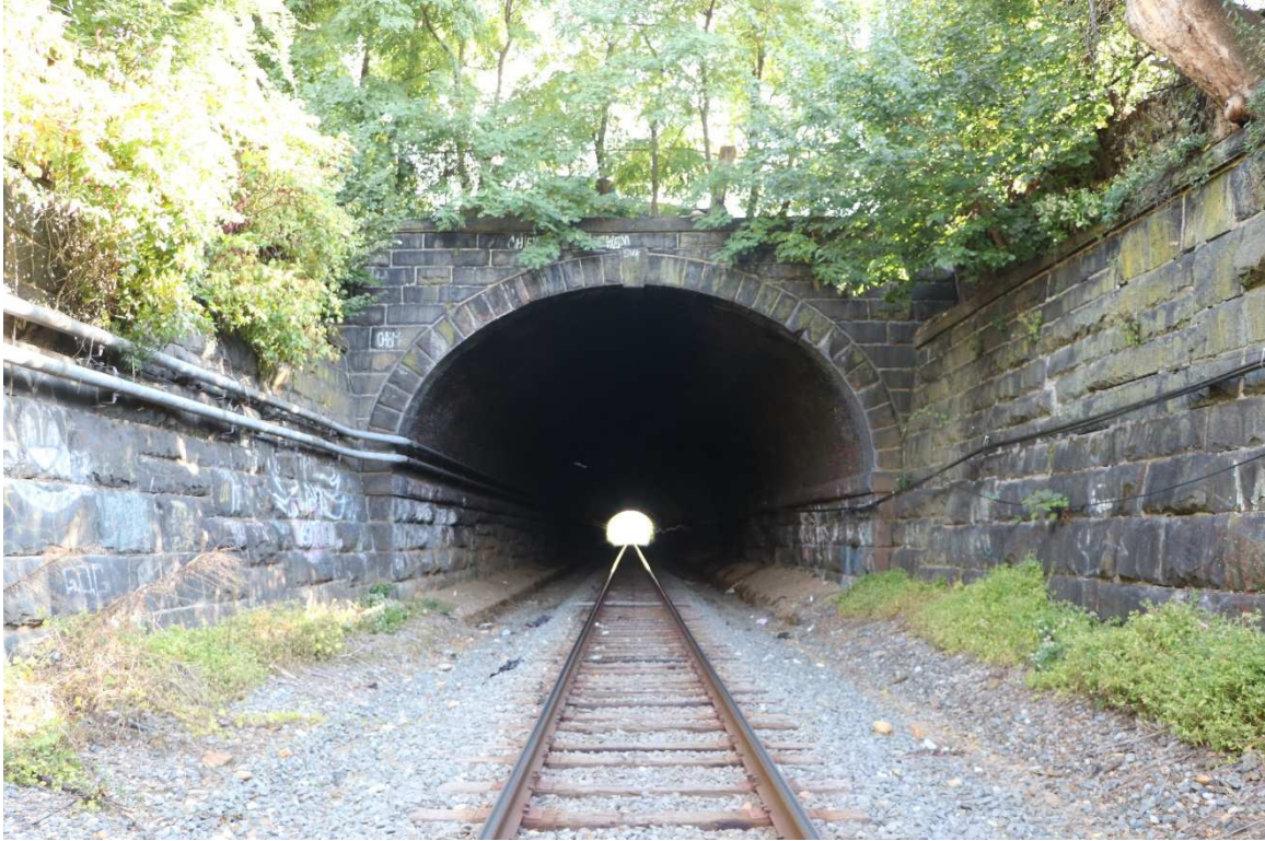
Photograph #7: Boone Tunnel southwest portal and retaining walls, looking northeast. October 15, 2021.
