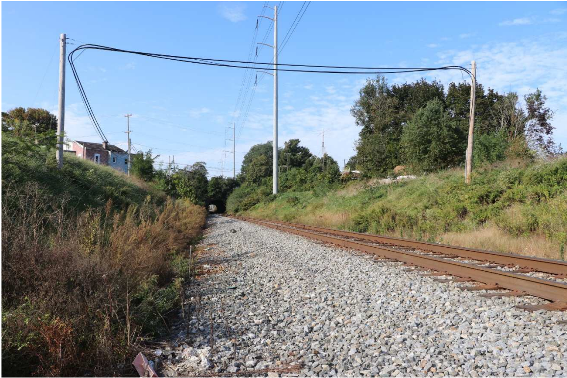
Photograph #1: Boone Tunnel northeast portal, tracks, and setting, looking southwest. October 15, 2021.
