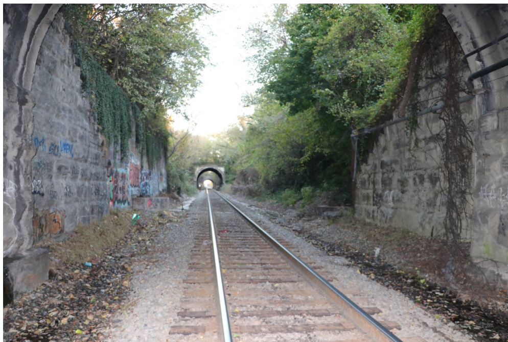
Photo 4: Eastern abutments, looking east to Barclay Street
