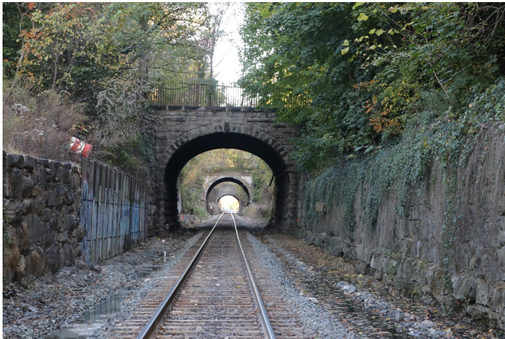
Photo 1: West portal and track, looking east to Barclay Street
