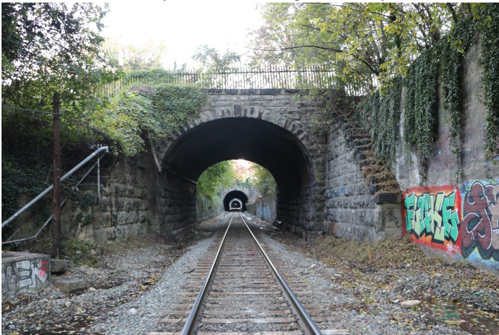
Photo 2: East portal, looking west to Calvert Street
