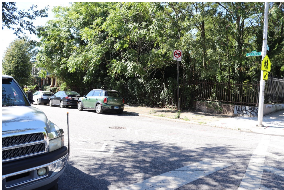
Photo 6: Guilford Avenue over CSX tracks, looking southwest
