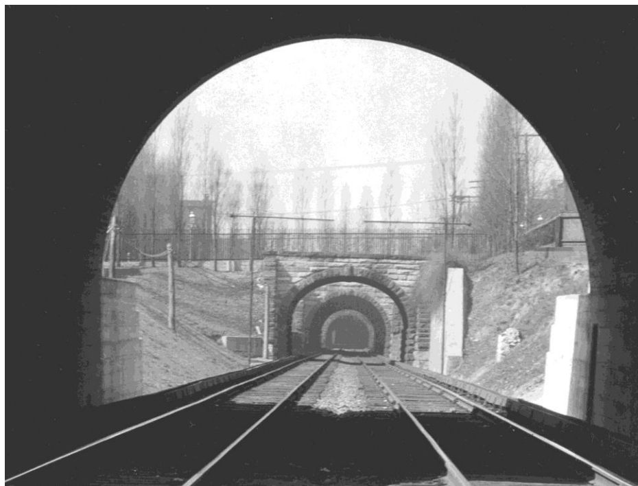
Figure 4: East portal of the Guilford Avenue Bridge, looking west from the Barclay Street Bridge, circa 1925. Image Credit: B&O Railroad Historical Society
