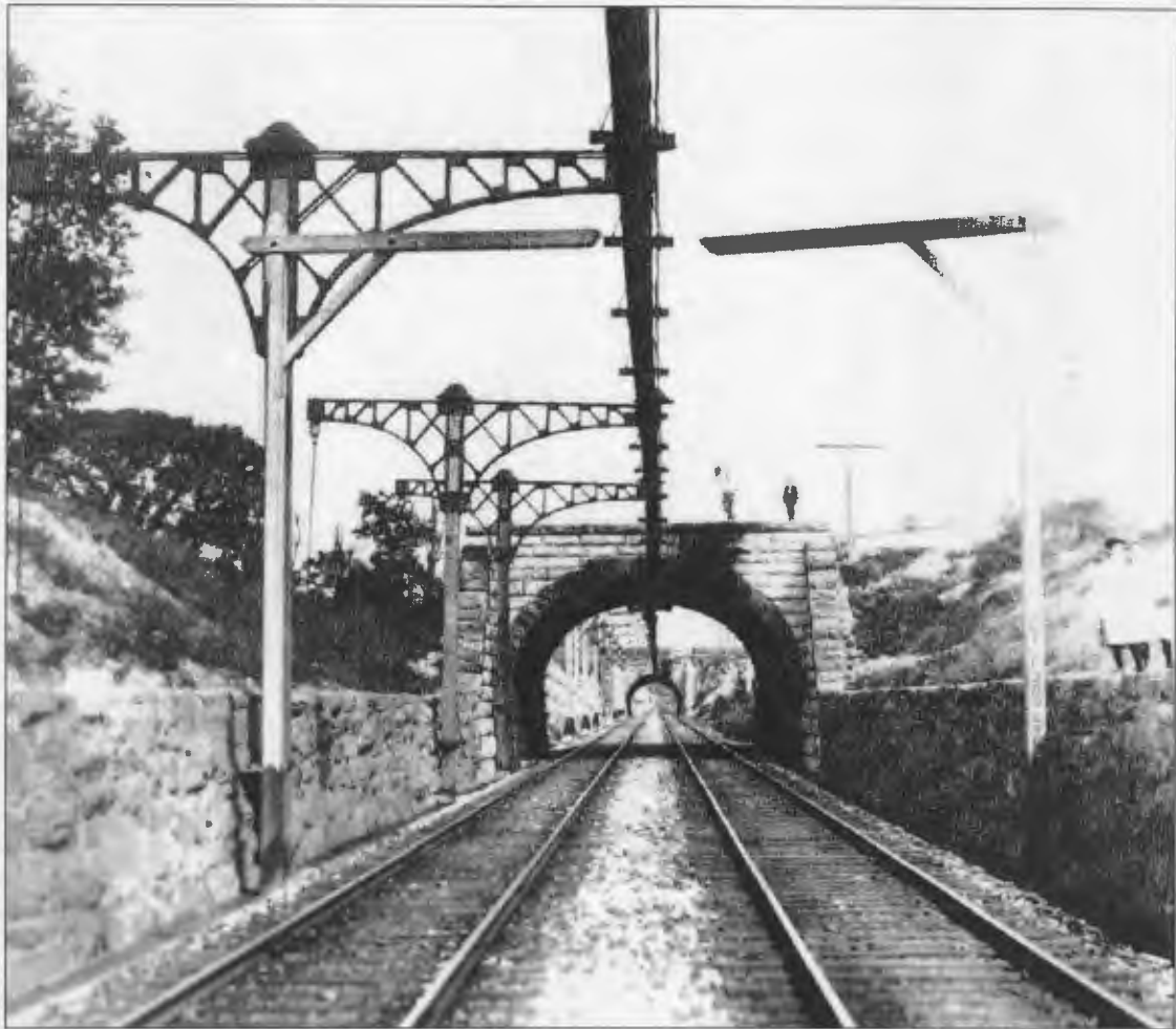
Figure 2. Circa-1901 View of the B&O Railroad Baltimore Belt Line's Overhead Third-Rail System, Looking towards the Guilford Avenue Tunnel (Smithsonian Institution Collection 1901).
