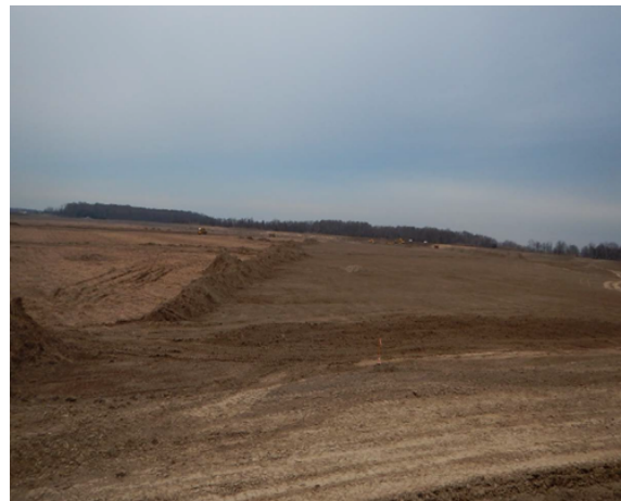
Construction activities in the Pearce Creek DMCF Photo Credit: Sealaska Constructors, LLC
