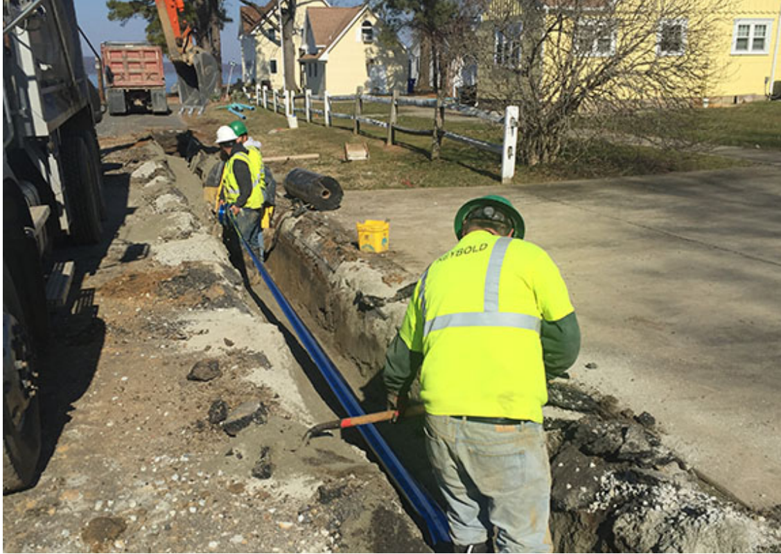
The waterline being installed within the communities. Photo: AECOM
