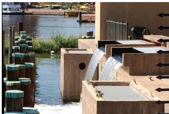
A geothermal heat sink at the World Trade Center provides oxygenated water to the harbor.
