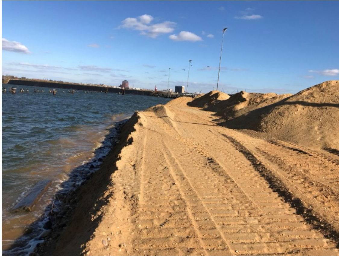
Earthen retaining walls called dikes are being raised to increase capacity at the Masonville Dredge Material Containment Facility
