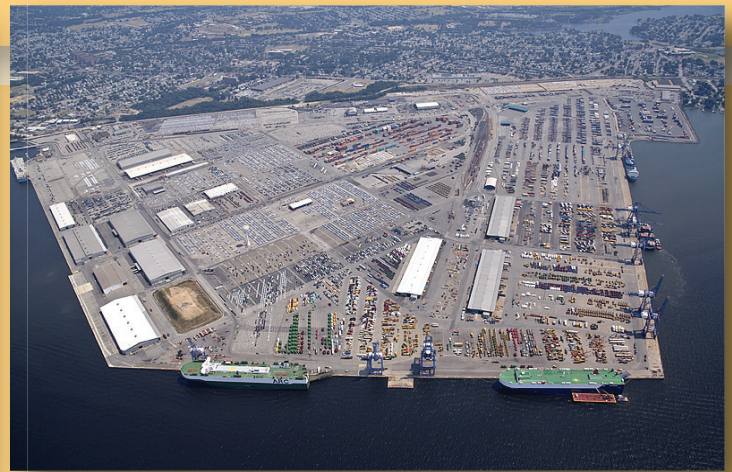
Dundalk Marine Terminal
